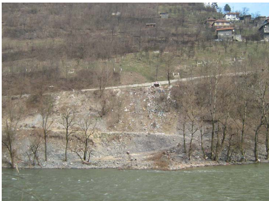
Figure 36. The current state of the hillside on which the left block of the dam is planned to build
