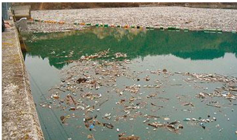
Figure 43. An example of waste accumulating in front of the dam
