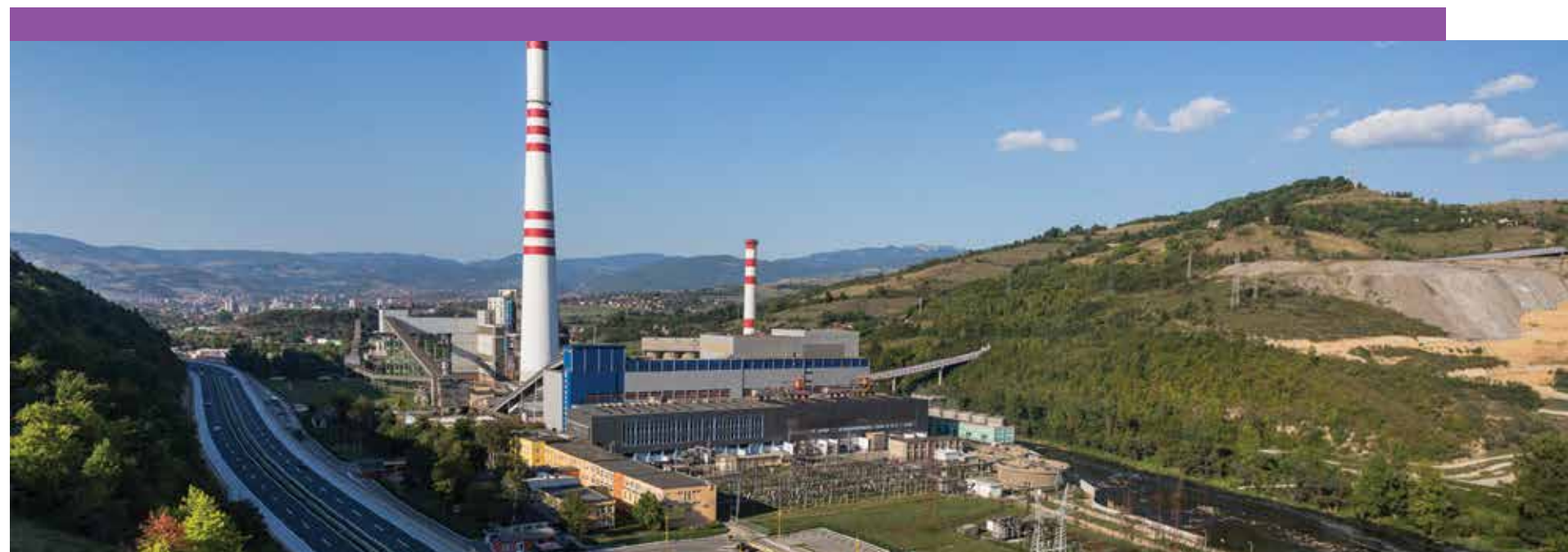
Thermal Power Plant Kakanj
