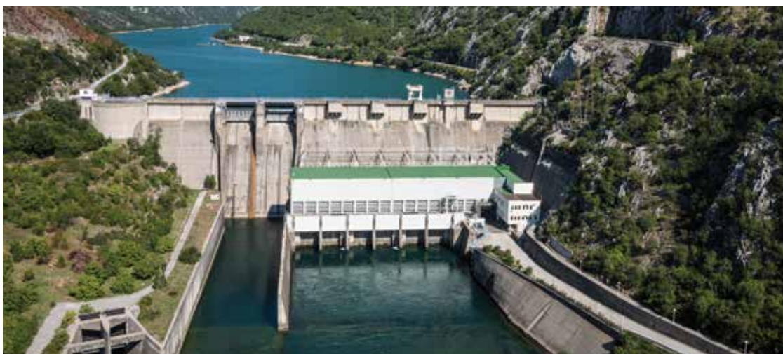
Hydro Power Plants on Neretva/ HPP Salakovac
