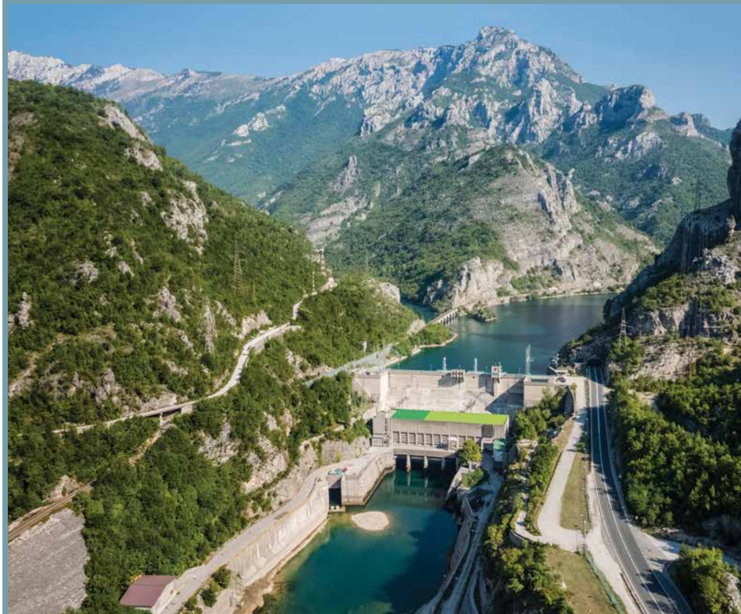
Hydro power plants on Neretva/ Hydro power plant Grabovica
